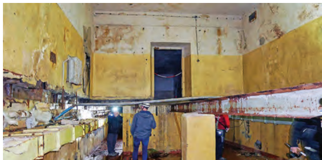
Koralle bunker; the missing floor shows the limited headroom below. Photo Vin Stenhouse
